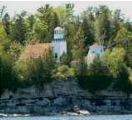
Sherwood Point Lighthouse
